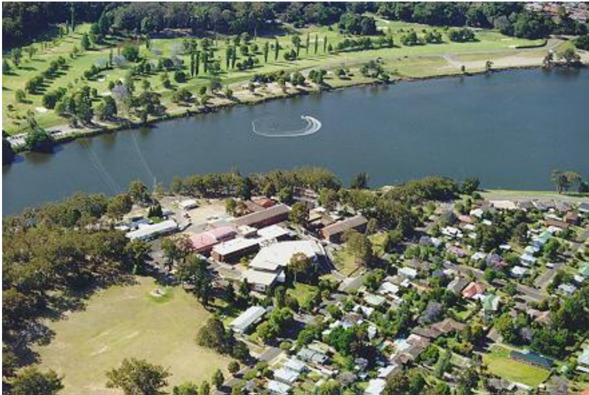
Figure 12 – Aerial view of Nowra District Memorial Hospital and Nowra Park, adjoining the Shoalhaven River, about 2010.
